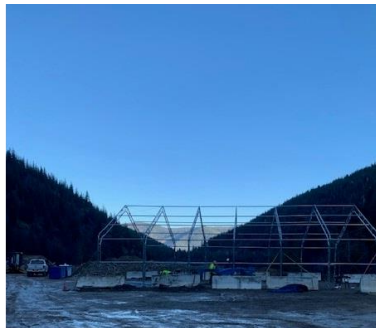
Shop Facility in construction
