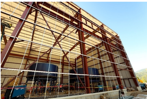
Figure 3: Tailing Thickener Tanks in place
