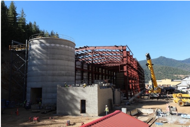
Figure 7: Processing Building looking north
