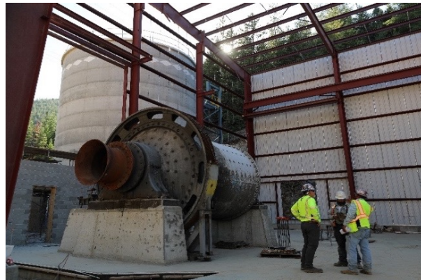
Figure 2: Refurbished Regrind Mill on its bearings
