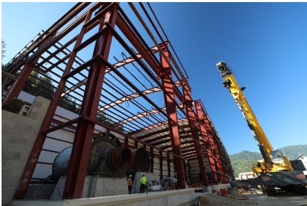
Figure 1: Primary Ball Mill and Regrind Mill
