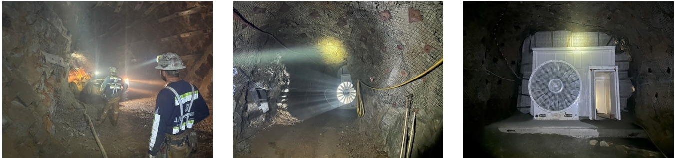
Figure 9: Ongoing Underground Development activity
