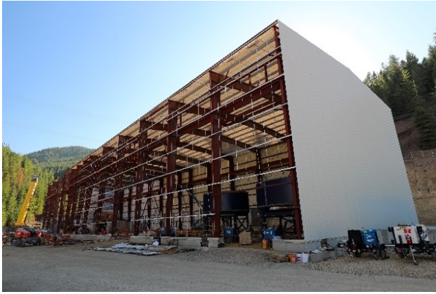
Figure 5: Processing Facility looking south
