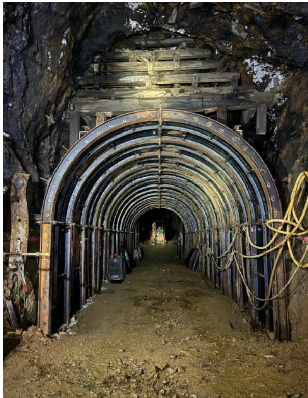
Figure 5: Steel Sets supporting ramp through Cate Fault
