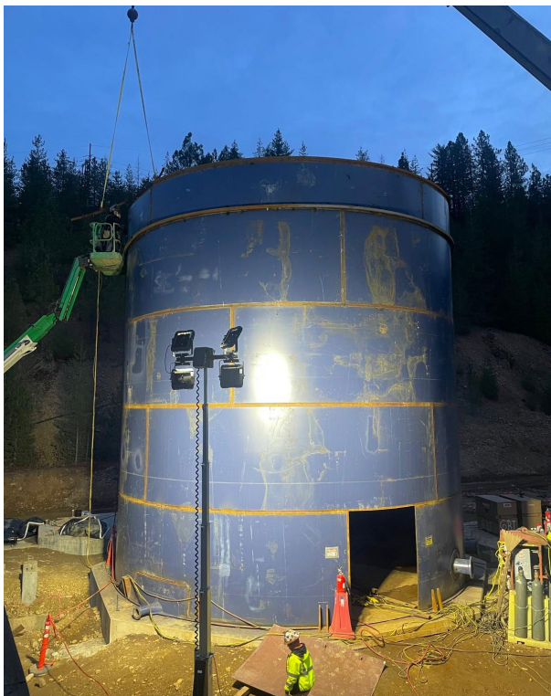
Figure 4: Tailings storage tank construction (December 2024)
