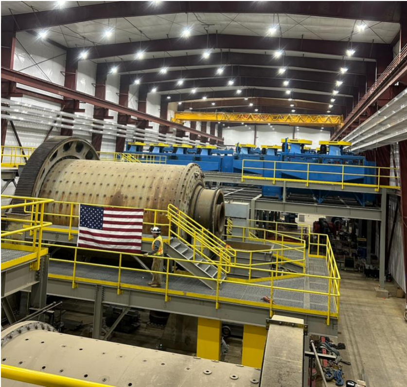
FIGURE 1: Refurbished flotation tanks from Teck's Pend Oreille Mine being inserted on their mezzanine floor
