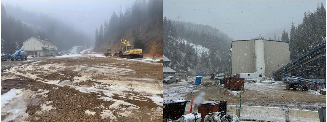
Figure 2: Progress in the main Kellogg yard from January 10, 2024, to January 10, 2025
