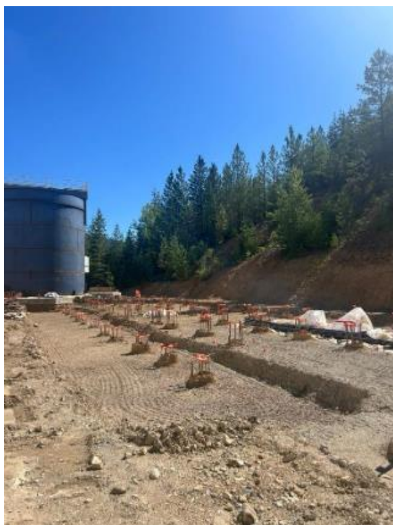
Figure 3 – Tailings Filter Press (42% complete) - foundations being prepared for concrete pour
