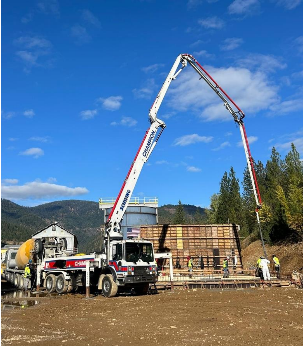
Figure 1: Filter Press Concrete Foundations in Progress
