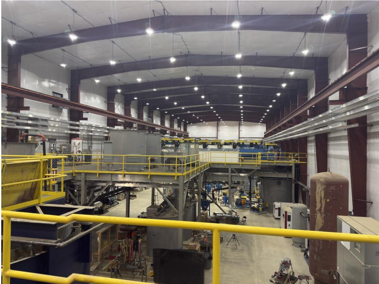
Figure 2: Processing Plant – Piping and Electrical Installation Advancing
