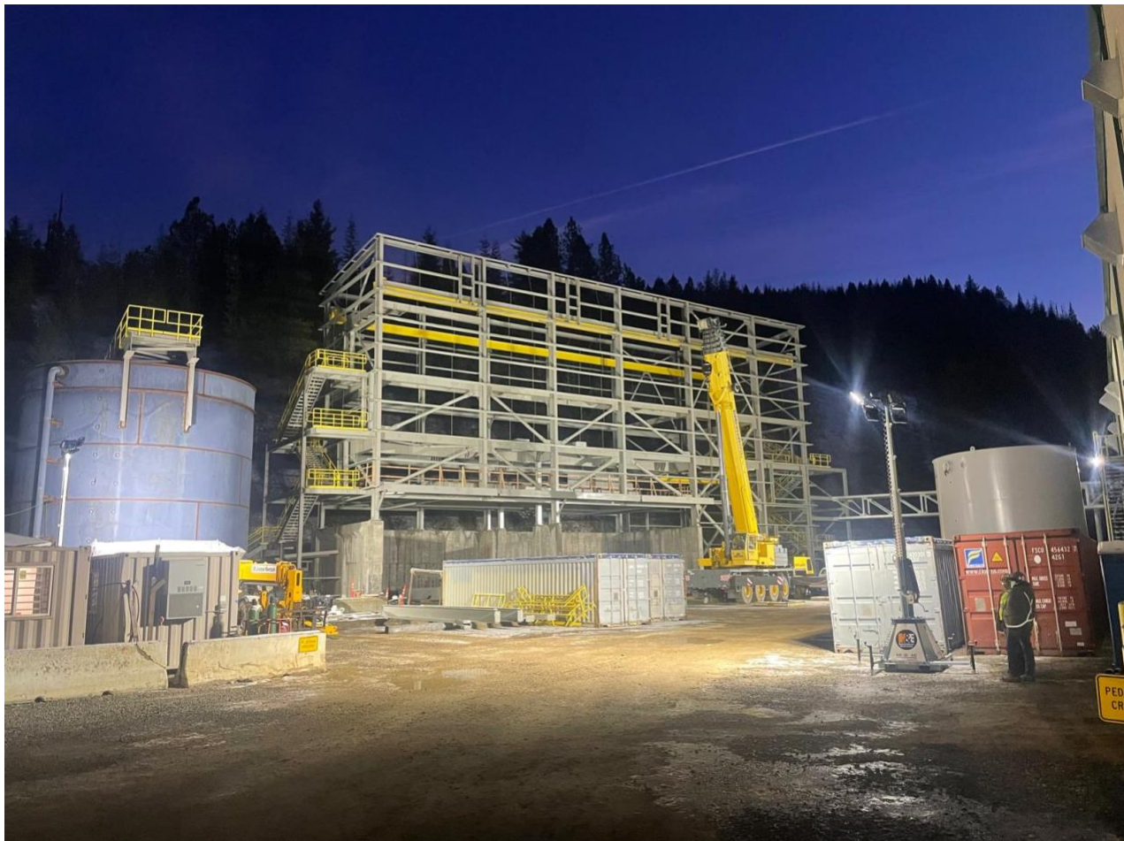
Figure 1. Tailings Filter Press Superstructure ready for installation of Metso's Filter Press
