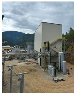
Tailings Filter Press Building
