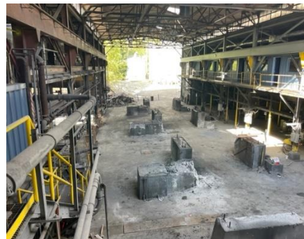
Photo 2: Pend Oreille mill building, following demobilization
