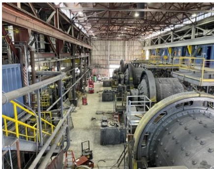
Photo 1: Pend Oreille mill building, prior to demobilization
