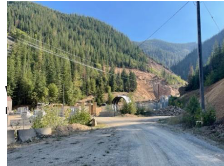
Overhead power installation
