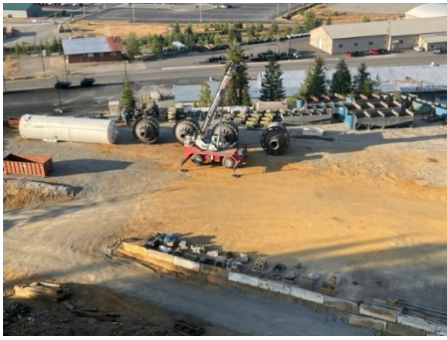
Ball mills, flotation cells and lime silo in BH yard
