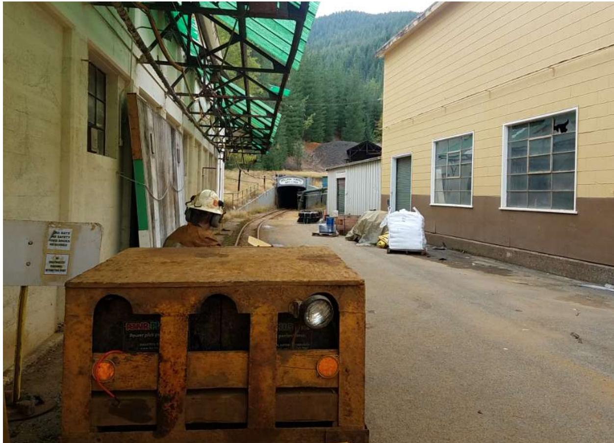
Figure 18-1 Kellogg Office Complex and Kellogg Tunnel Portal
