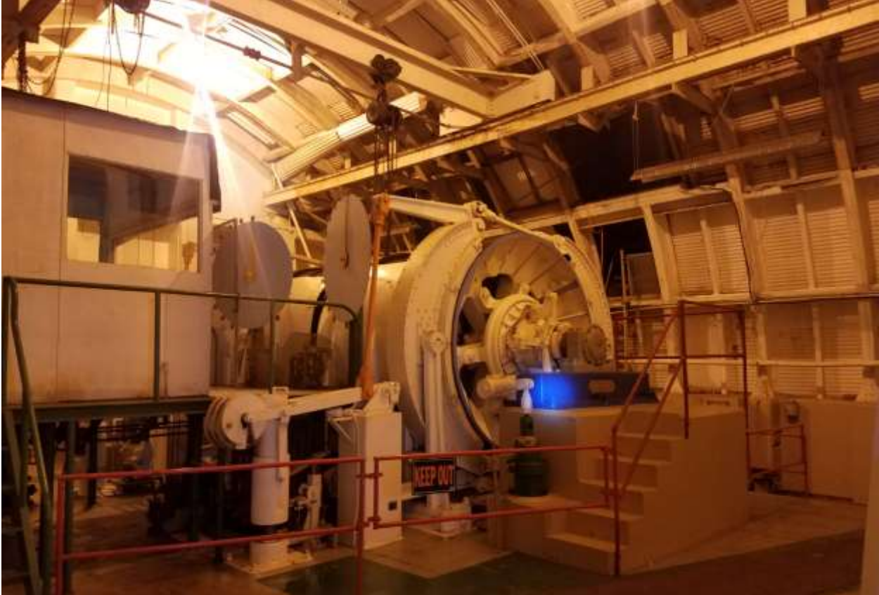
Figure 18-8 #2 Shaft Double Drum Hoist Room
