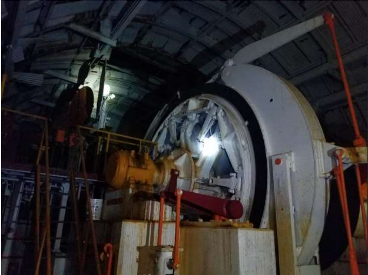
Figure 18-3 #1 Hoist and Hoist Room 9-Level
