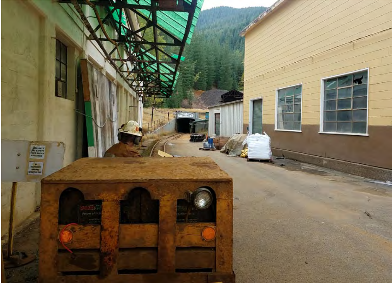
Figure 18-1 Kellogg Office Complex and Kellogg Tunnel Portal
