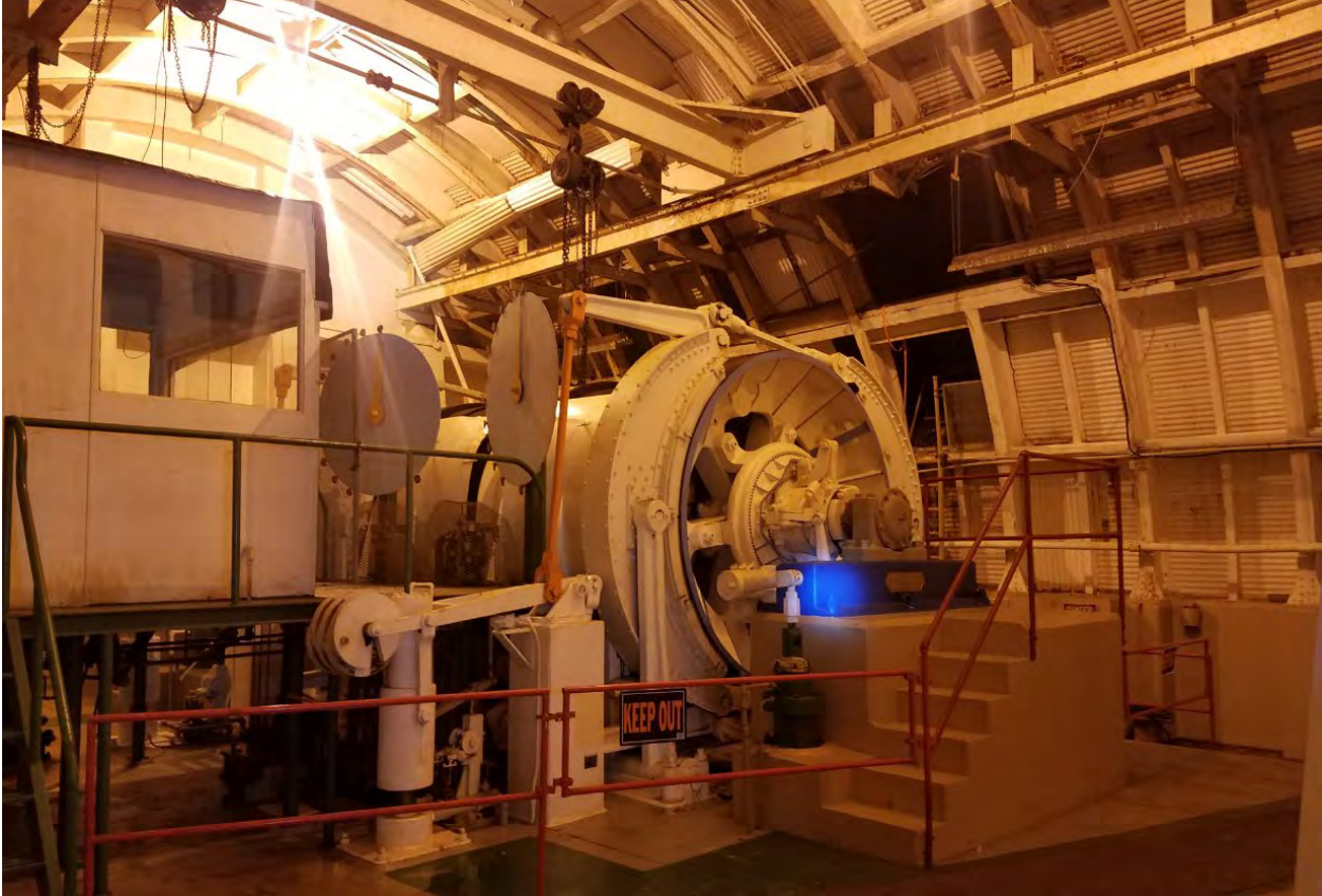
Figure 18-8 #2 Shaft Double Drum Hoist Room
