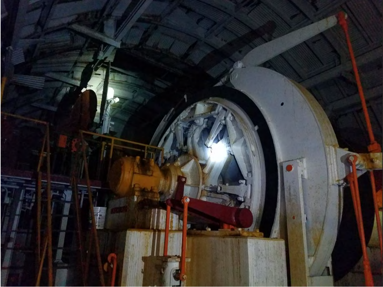
Figure 18-3 #1 Hoist and Hoist Room 9-Level
